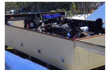
Building 9 at full Capacity
